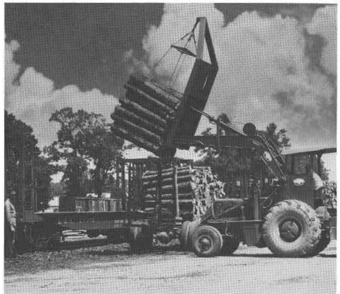
Later, logs and pulpwood were loaded with power equipment.
